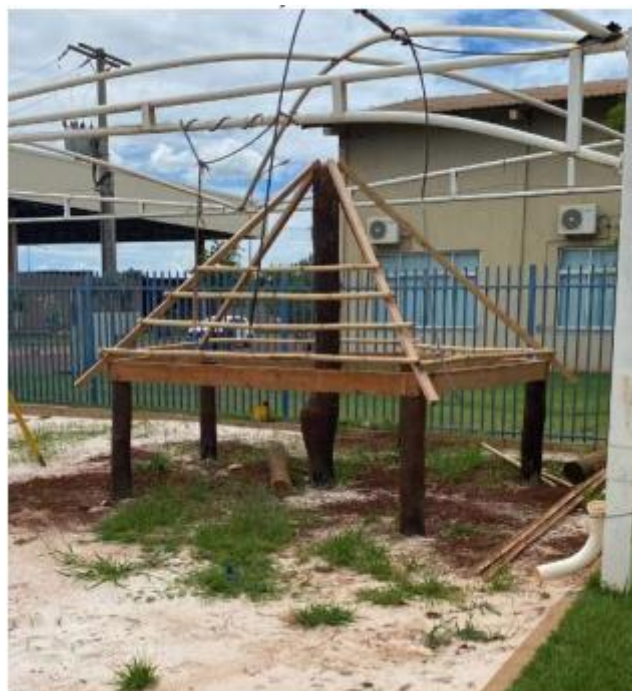
Figure 11. Detail of the execution of the oca roof structure.
