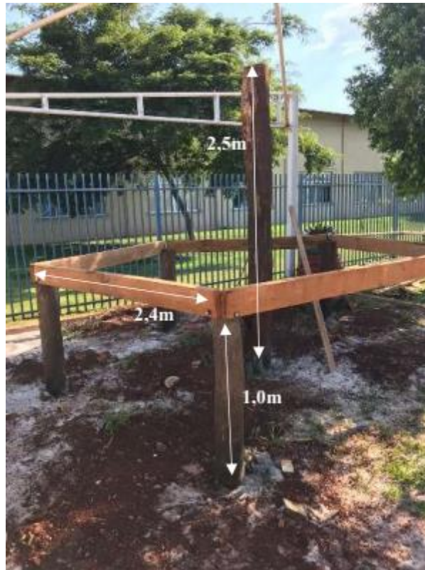
Figure 10. Detail of the execution of the oca pillars.
