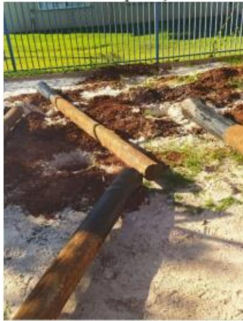
Figure 9. Pillars with asphalt paint application.
