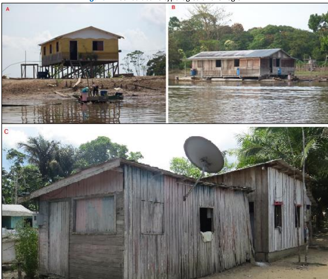
Figure 1: Constructive typologies of the region.
