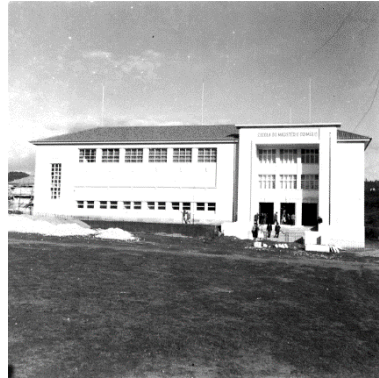
Figure 3 - Visit to the construction site of EMPC
